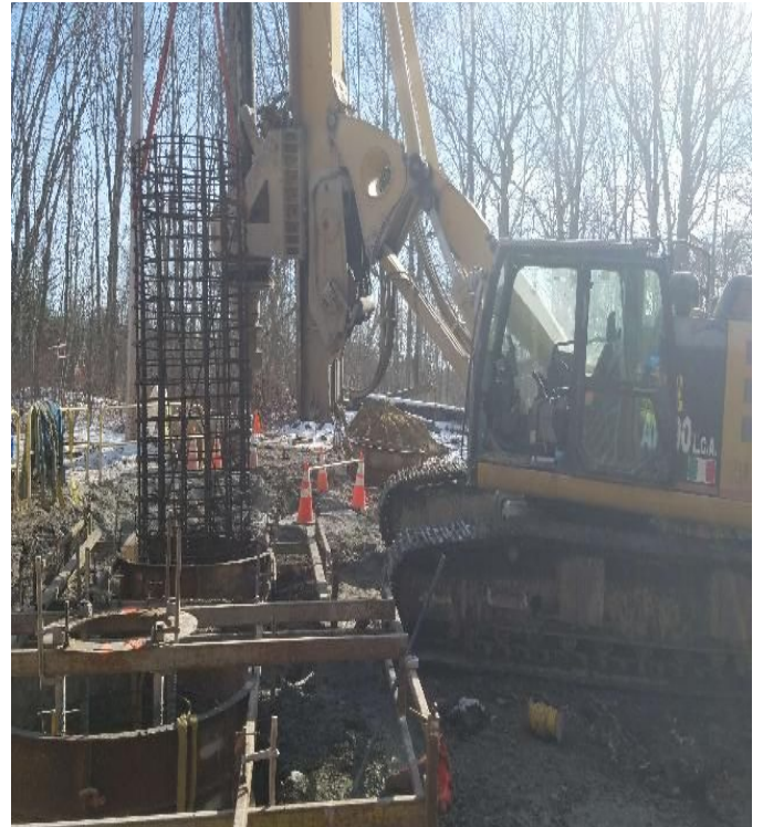
Fig 16: MJ prepping to pour foundations for Str. 58. Viewing south. (02-12-20).
