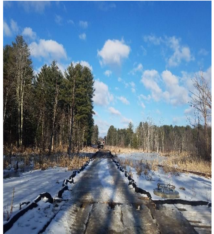
Fig 14: Building access road from Str. 116 to Str. 114. Through wetlands NW11 and NW13. Viewing north. (02-12-20).
