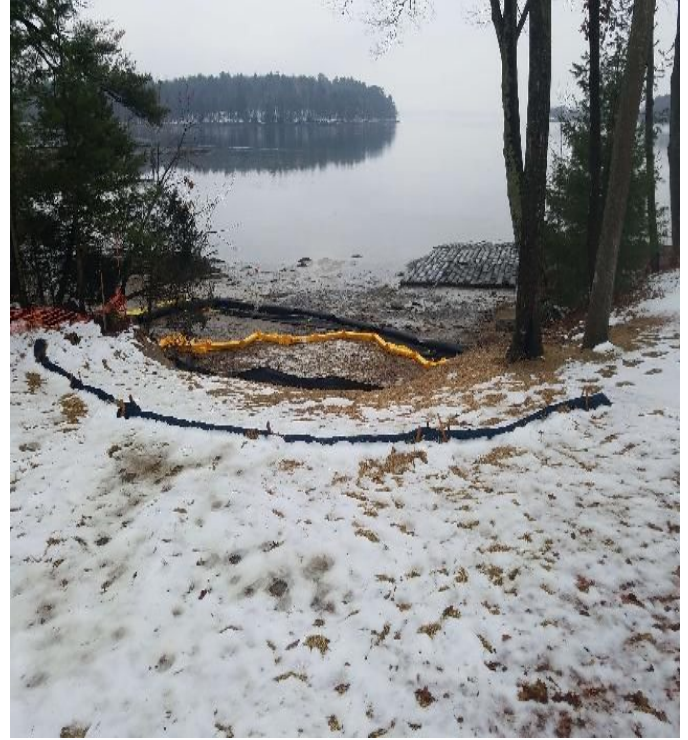
Fig 10: Turbidity barrier remains in place in intertidal zone at Gundalow landing/east side of the Bay. Viewing southwest. (02-11-20).
