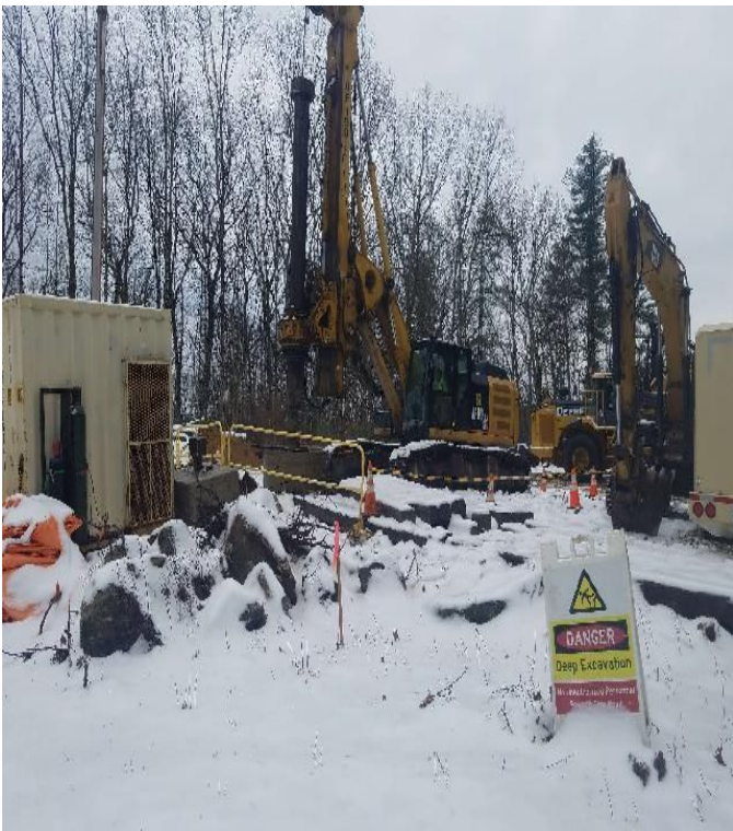
Fig 7: Crew continues to drill at Str. 58. Viewing south. (02-10-20).
