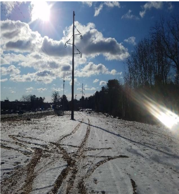
Fig 15: Strs. 123 and 124. Viewing south. (02-12-20).
