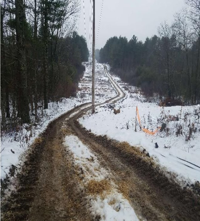
Fig 9: Access road between Strs. 57 and 58. Viewing west. (02-11-20).
